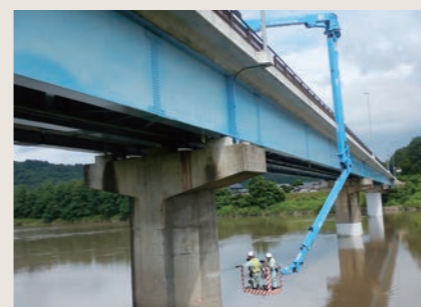
橋梁点検 (西倉橋)
