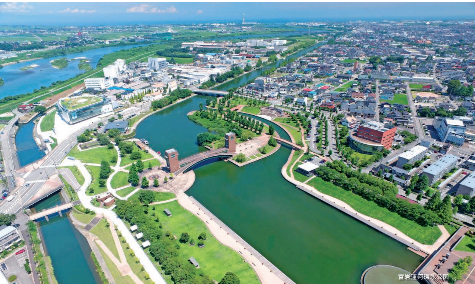
Fugan Canal, the Beginning of Urban Planning for Toyama City
